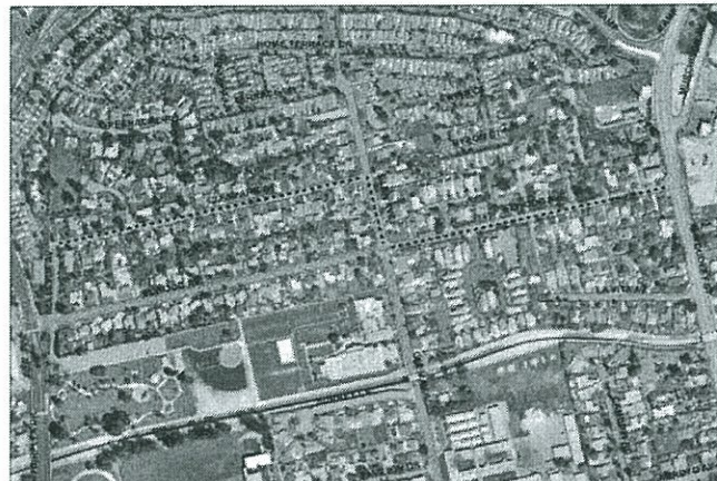
Sidewalks - Elwood Avenue and Glenpark Street
