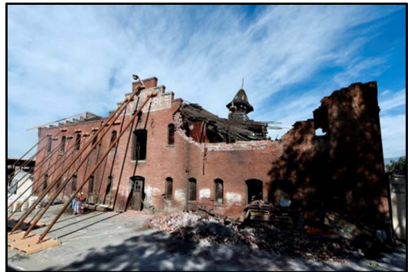
Current City Stable Facility
