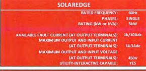
NOMINAL ESS AC VOLTAGE MAXIMUM ESS DC VOLTAGE: 450V AVAIJABLE FAULT CURRENT DERIVED FROM THE ESS: DATE CALCUALTION WAS PERFORMED:
