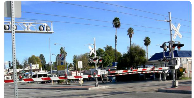
Photo of a four-quadrant gate crossing. Four gate crossing arms will span over all lanes of traffic to prevent vehicles from around the gates when the arms are lowered and not waiting for a train to pass before entering the crossing.
