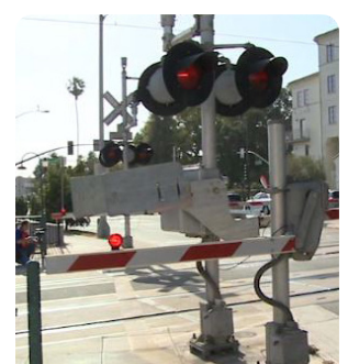
Pedestrian gate arms are lowered simultaneously with the quadrant gate arms along the street, when a train is approaching. This combination of arms will stop all traffic from crossing the tracks including pedestrians and cyclists.
