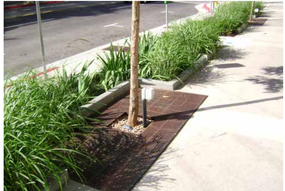
Flow-through planters collect stormwater and filter sediment and pollutants
