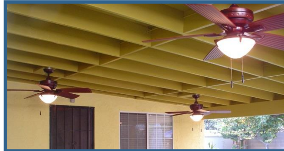
Repaired Patio Cover
