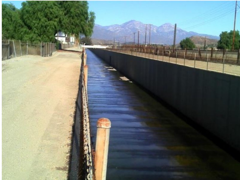
ESGV_SJC_DS Looking Upstream
