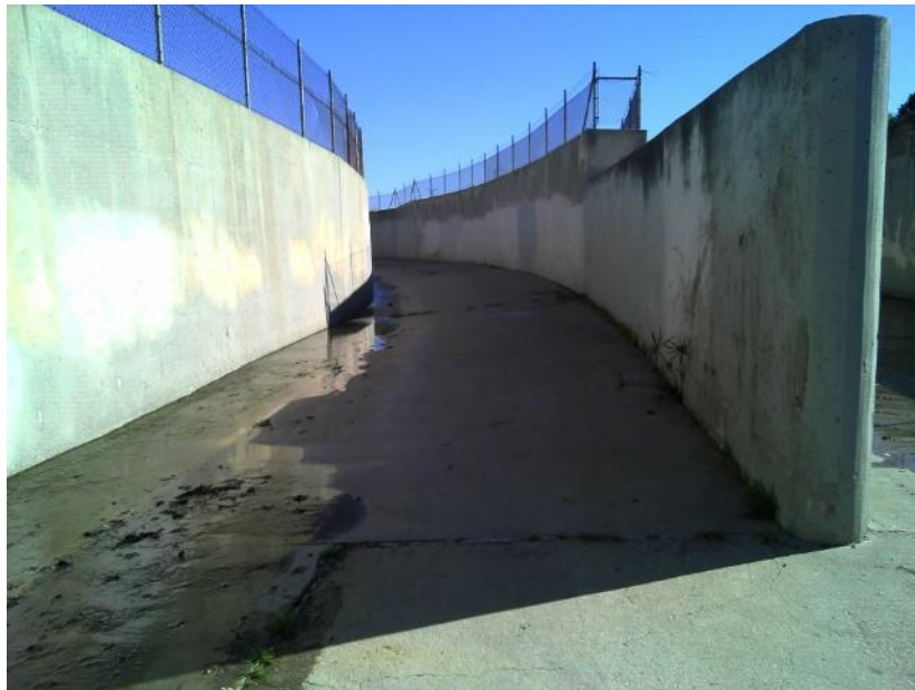
ESGV_LOW_DS Marshall Creek Flow Monitoring Location Looking Upstream
